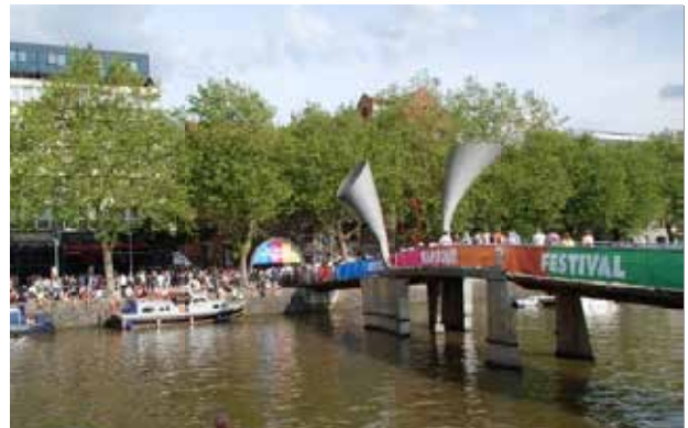
Bridge in Bristol Harbourside
